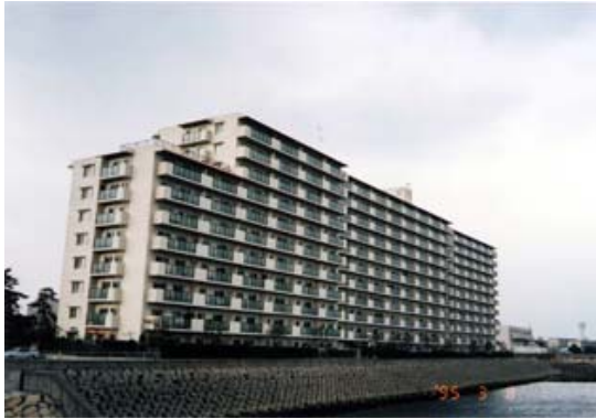
Figure 1. Photograph showing overall view of the building looking from the west side, with blocks A, B and C from left to right, where the damage to quay wall to the west can be noticed.
